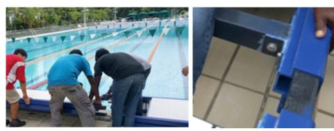
Figure A: Connecting the EndWall sections together with the Connector Sleeves (image on right).
