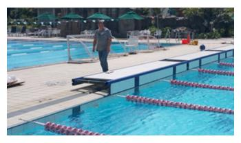
Figure C:The EndWall sections are assembled and connected together on the pool deck.
